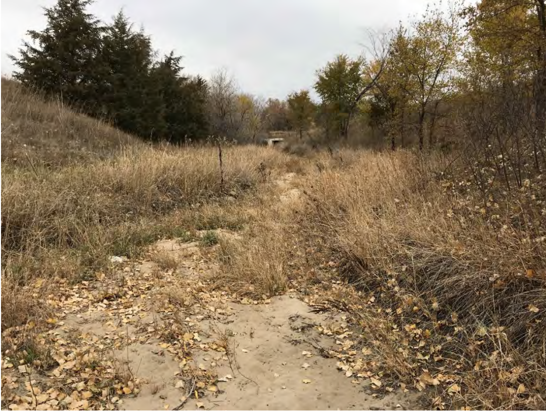
Figure 47. Vegetated channel in Segment 7A
