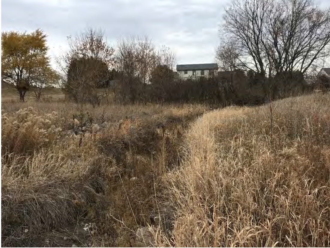
Figure 30. FEMA bank repair area in Segment 4B with established vegetation
