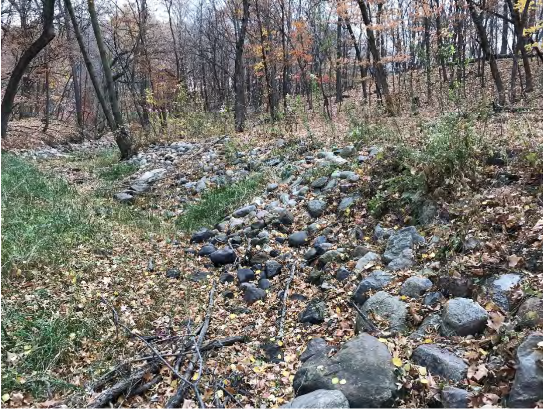
Figure 17. Bank stabilization along the gravel road in the Kici Yapi reach
