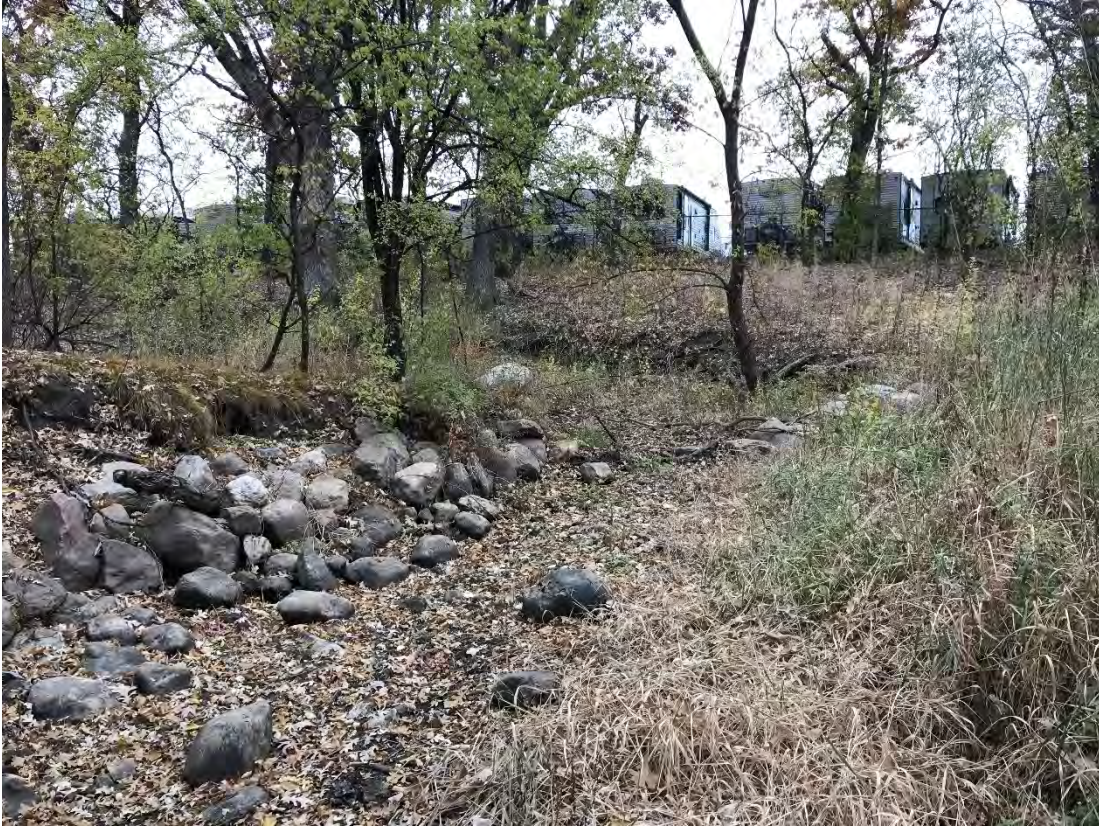
Figure 49. Former bank repair area and vegetation establishment in Segment 7B
