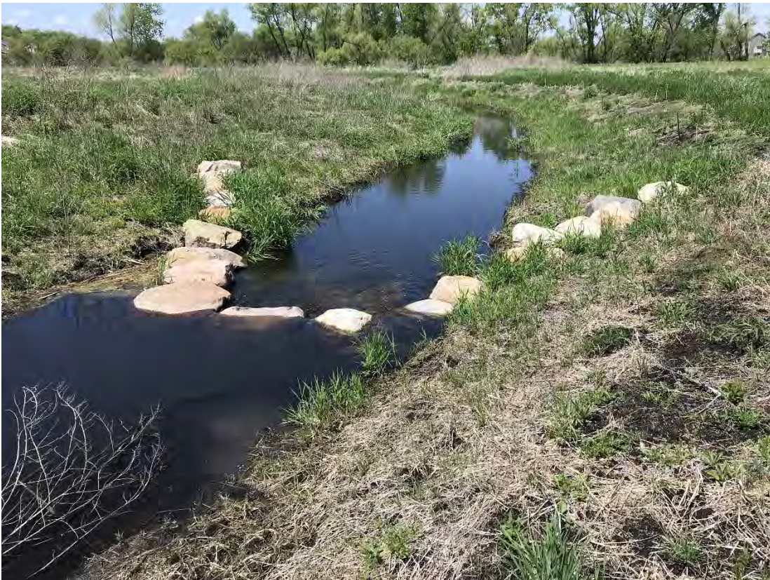
Figure 37. Boulder cross vane grade control installed in the new channel alignment in Segment 5B
