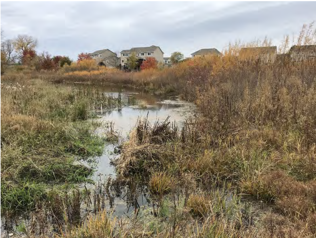
Figure 35. Equalized water levels in the west stormwater pond in Segment 5A
