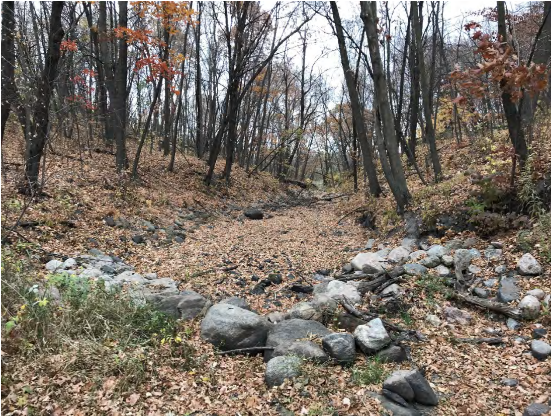
Figure 19. Rock cross vane in the Kici Yapi reach
