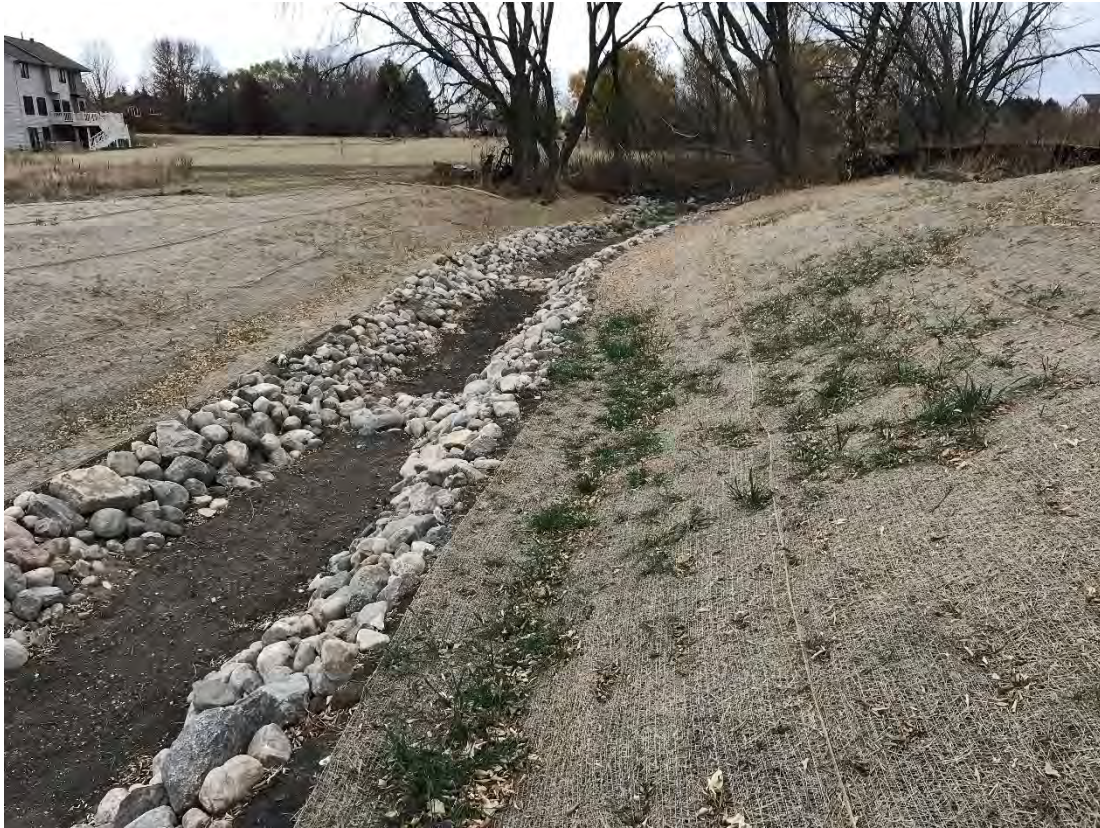
Figure 26. Repaired channel and floodplain benches downstream of the Gonyea culvert
