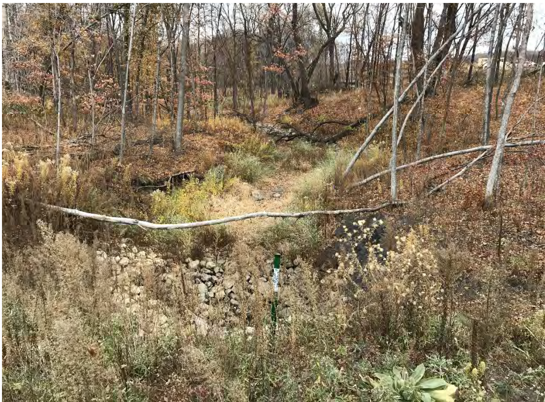
Figure 13. Open canopy and dense riparian vegetation downstream of Marsh Drive NE
