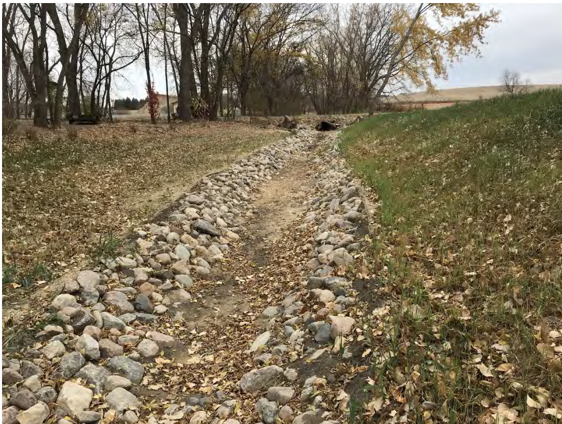
Figure 25. Repaired channel and floodplain bench upstream of Jackson Trail
