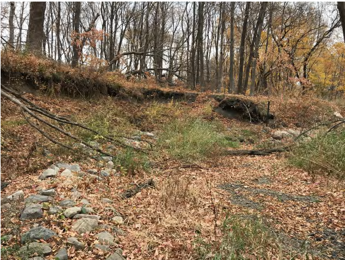
Figure 9. Boulder toe bank stabilization from the FEMA project
