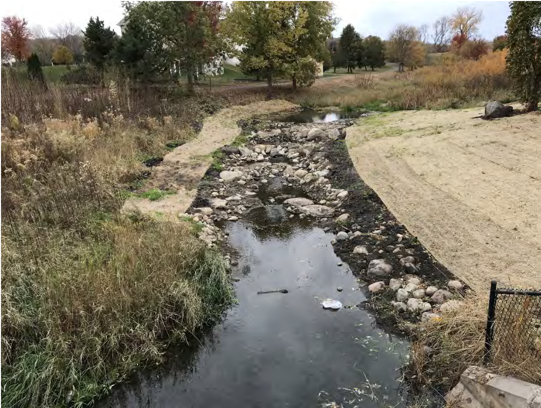
Figure 34. Boulder weirs installed upstream of Oak Ridge Trail in Segment 5A
