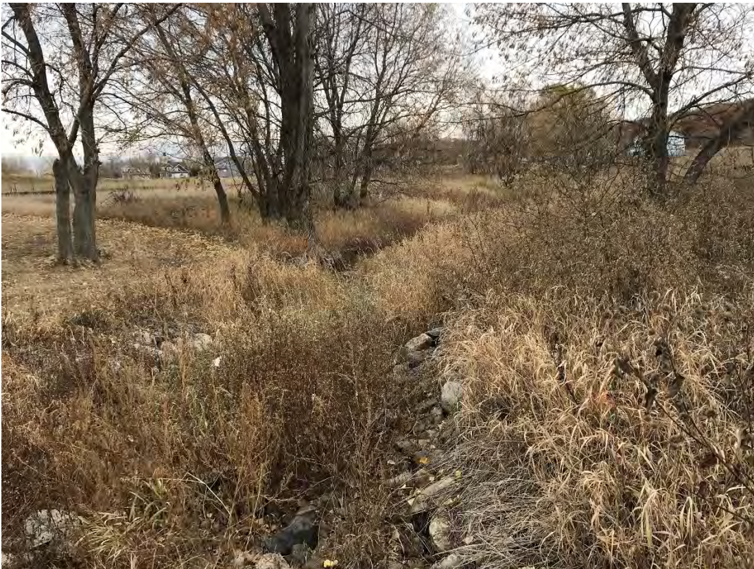
Figure 29. FEMA bank repair area in Segment 4B with established vegetation
