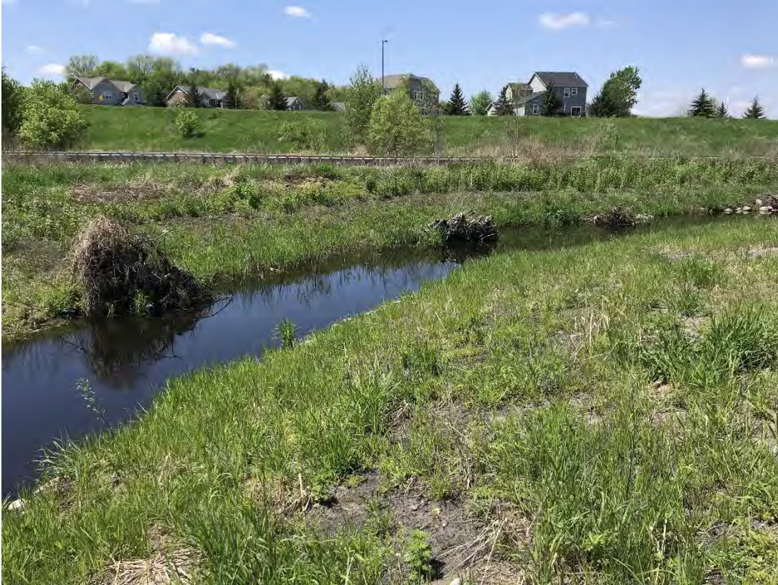
Figure 38. Rootwads installed along the new channel alignment in Segment 5B
