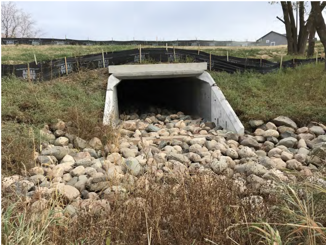
Figure 31. New box culvert and road crossing in Segment 4B
