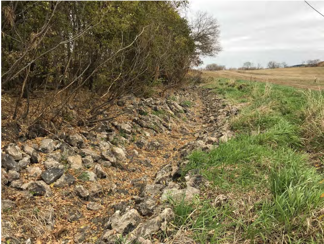
Figure 24. Repaired boulder toe downstream of Pike Lake Trail
