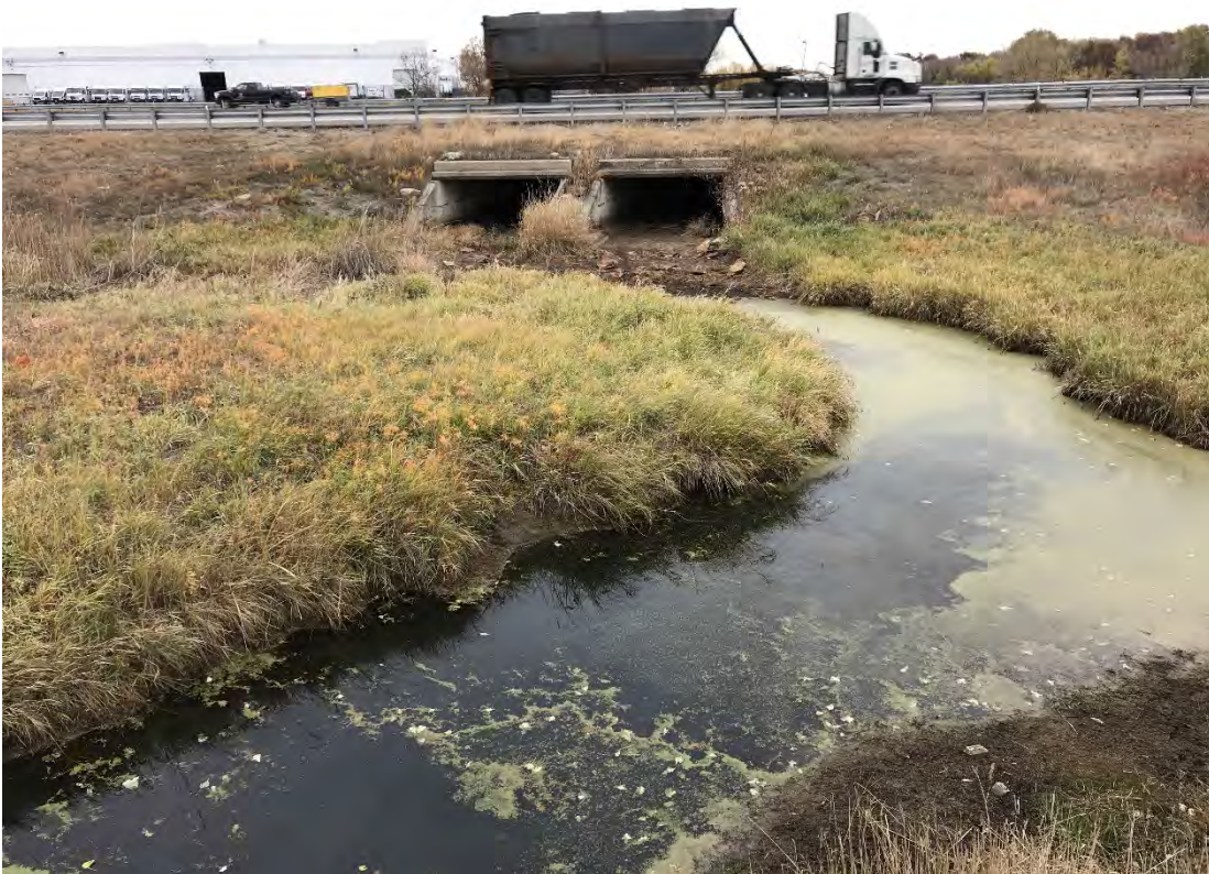
Figure 45. Stable, vegetated stream banks upstream of Highway 169
