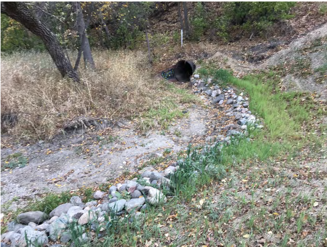
Figure 2. Bank repair upstream of Fountain Hills Road walking trail
