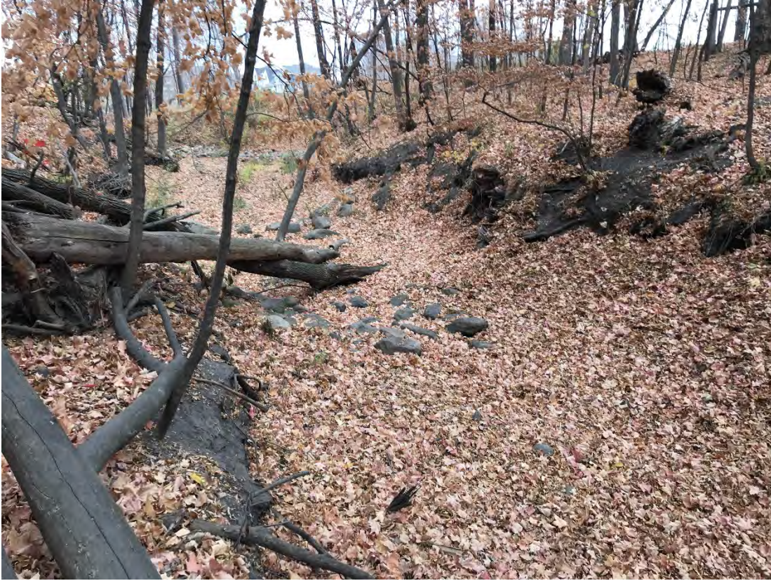
Figure 8. Boulder toe and cross vanes from the FEMA project
