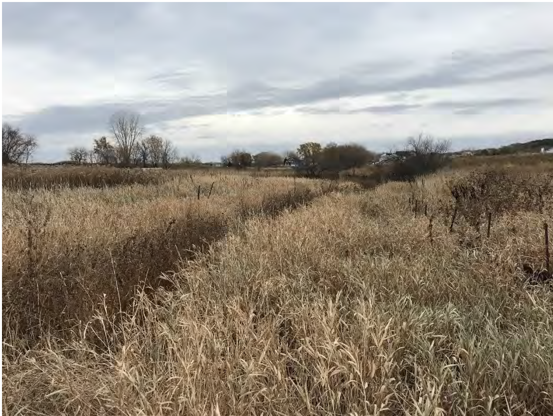
Figure 27. Dense vegetation within the PLOC channel in Segment 4A
