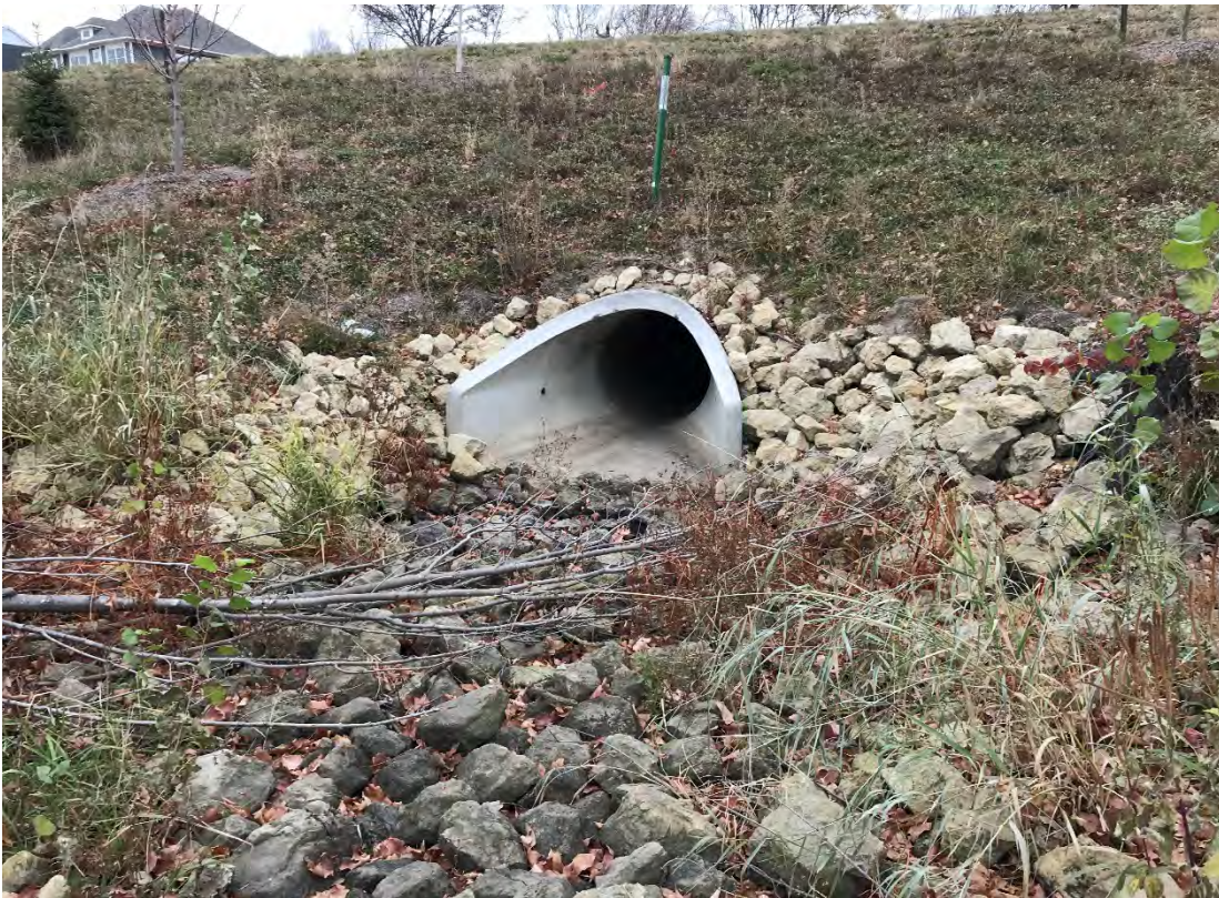
Figure 11. New culvert installed for a new road crossing (Marsh Drive NE)
