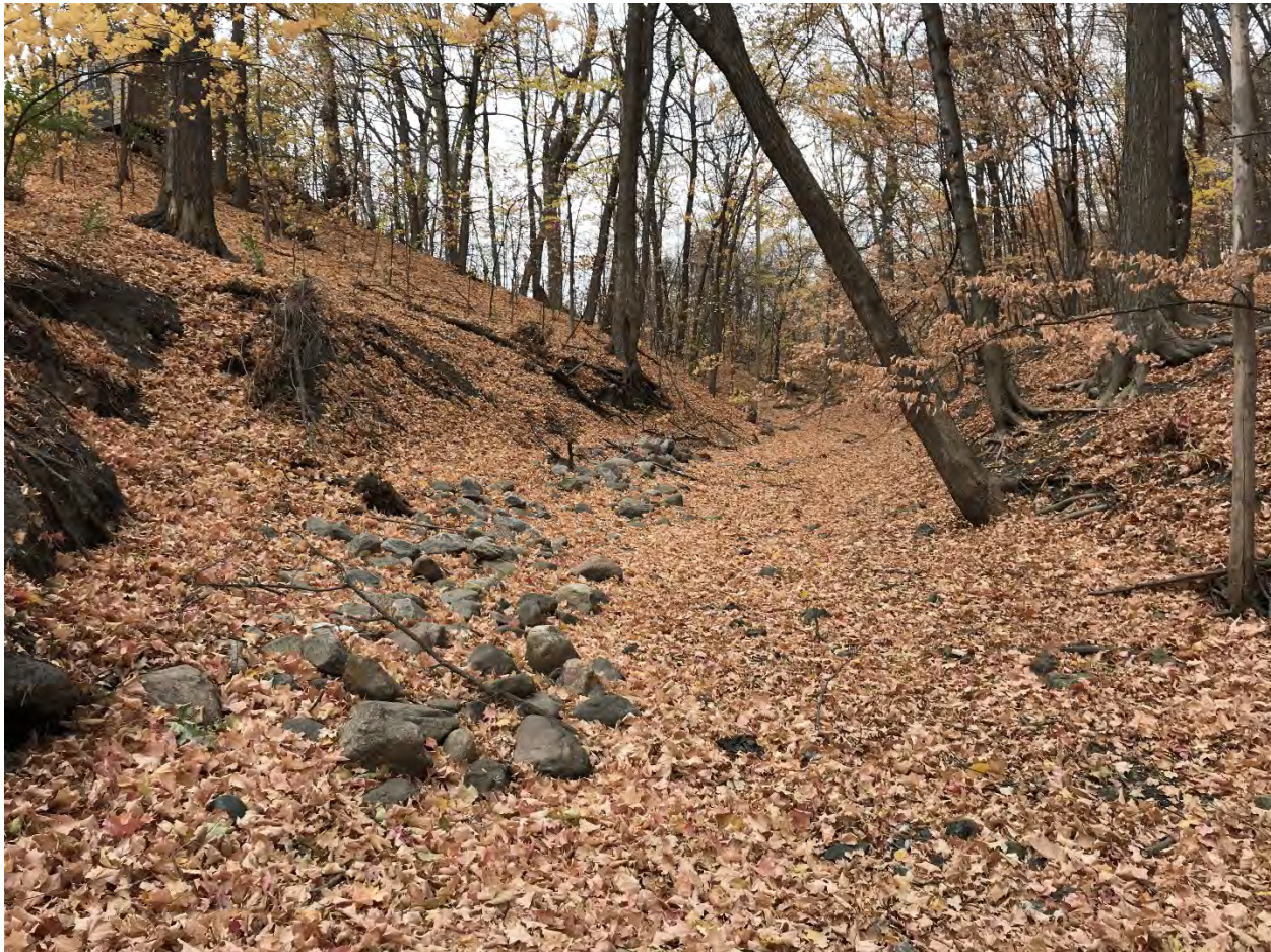
Figure 7. Boulder toe bank stabilization from the FEMA project
