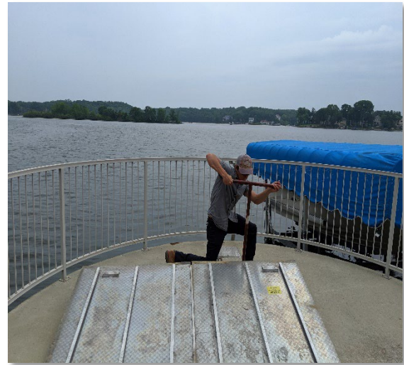
FIGURE 3 - OPENING THE LOW-FLOW GATE
