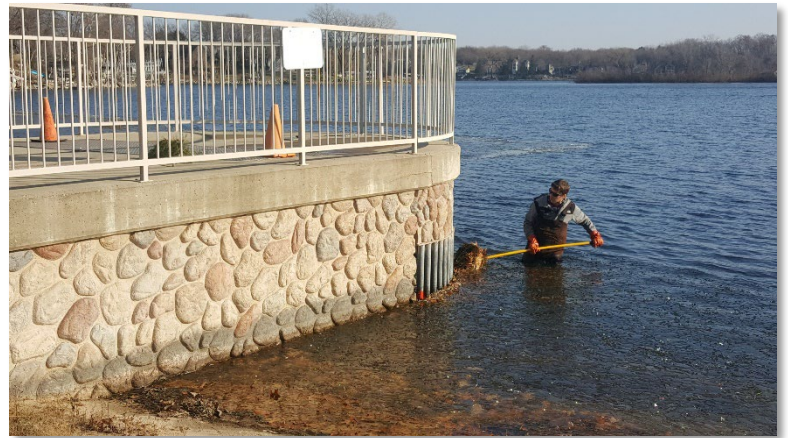
FIGURE 2 - REMOVING VEGETATION FROM OUTLET STRUCTURE
