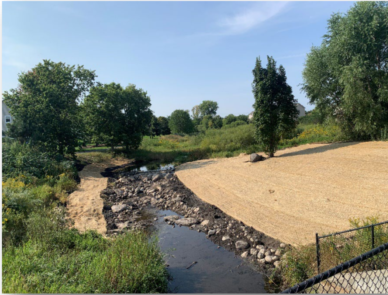
FIGURE 8 SEGMENT 5A STABILIZATION
