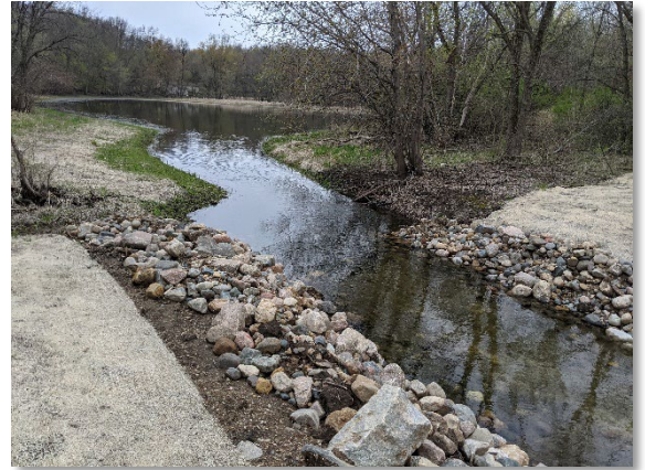
FIGURE 7 - STRAUSS DRIVEWAY AND CULVERT REMOVAL IN 2021
