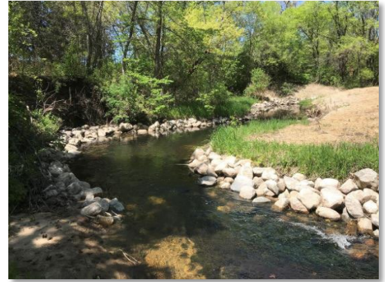
FIGURE 11 - BOULDER TOE BANK STABILIZATION IN SEGMENT 7A
