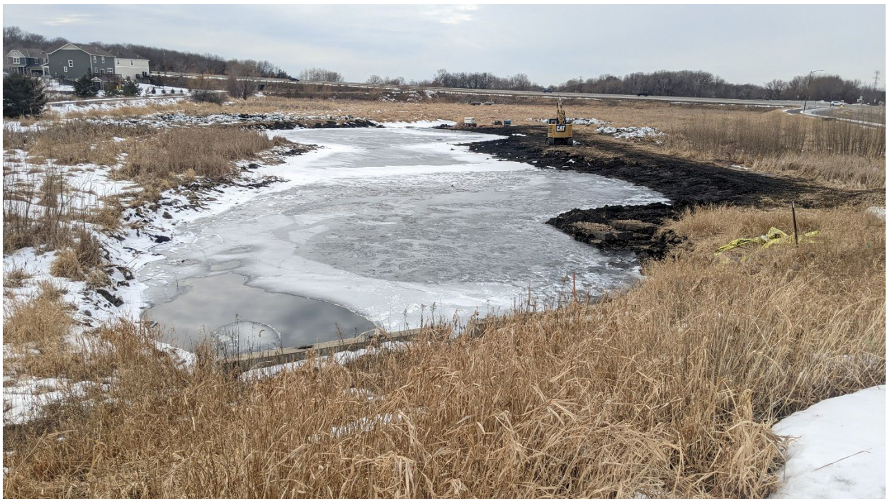
FIGURE 9 PIKE LAKE ROAD POND SEDIMENT REMOVAL
