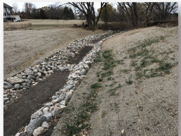
FIGURE 6 - SEGMENT 4 RESTORATION IN 2022
