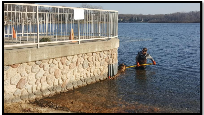
FIGURE 2 REMOVING VEGETATION FROM OUTLET STRUCTURE
