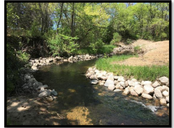
FIGURE 8 BOULDER TOE BANK STABILIZATION IN SEGMENT 7A
