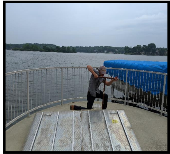
FIGURE 3 – OPENING THE LOW-FLOW GATE
