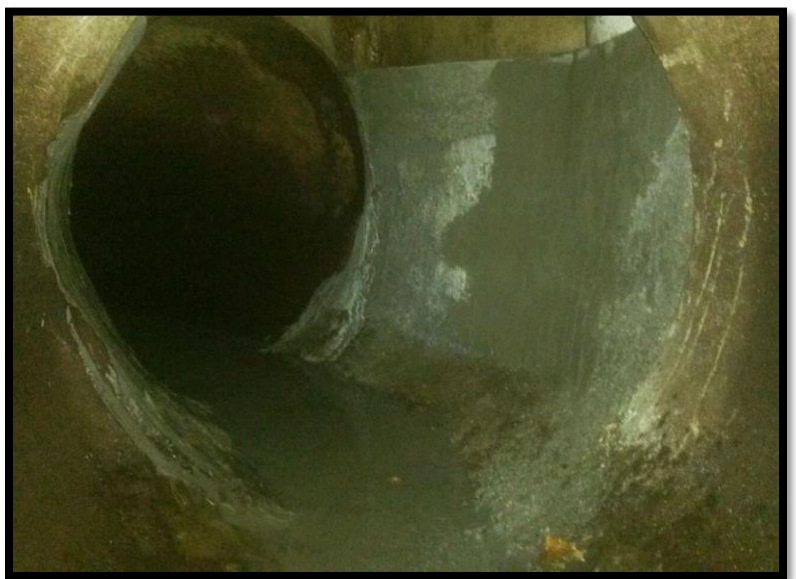
FIGURE 6 MANHOLE BENCH AFTER SMOOTHING
