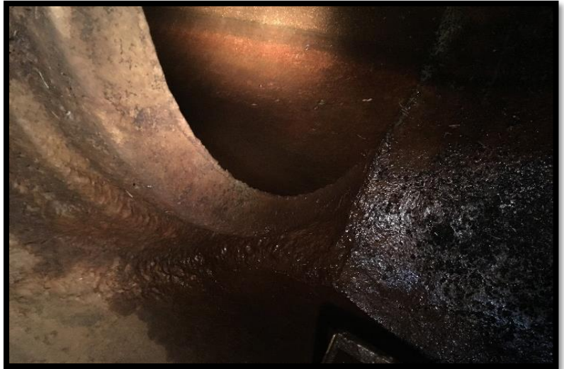
FIGURE 5 MANHOLE BENCH BEFORE SMOOTHING
