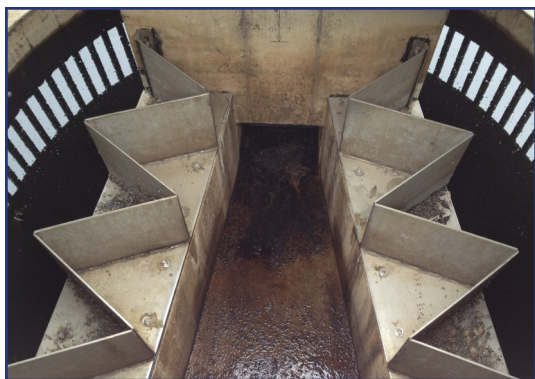
A look at the accordion-shaped fixed crest weir located inside the outlet structure on Prior Lake.
