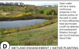
Open water presence in the central portion of the park in order o more effectively treat stormwater runoff via detentio and subsequent filtration through the Iron-Enhanced
