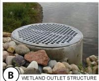
The wetland enhancement and outlet structure will hold back water in the wetland and will slowly release Enhanced Sand Filter for further
