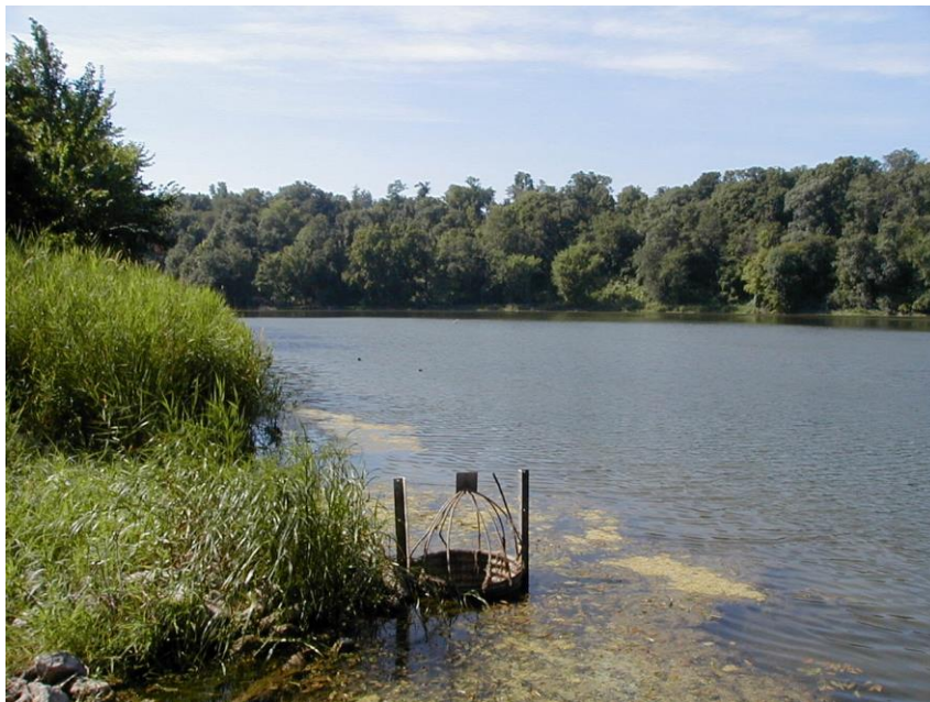
One of three outlet structures on Upper Jeffers Pond Segment 1. Note inefficient structure particularly for floatable debris control.
