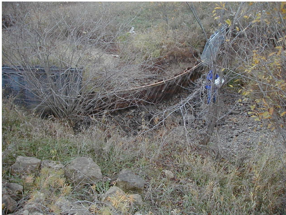
Sheet pile energy drop structure in poor condition Segment 7.
