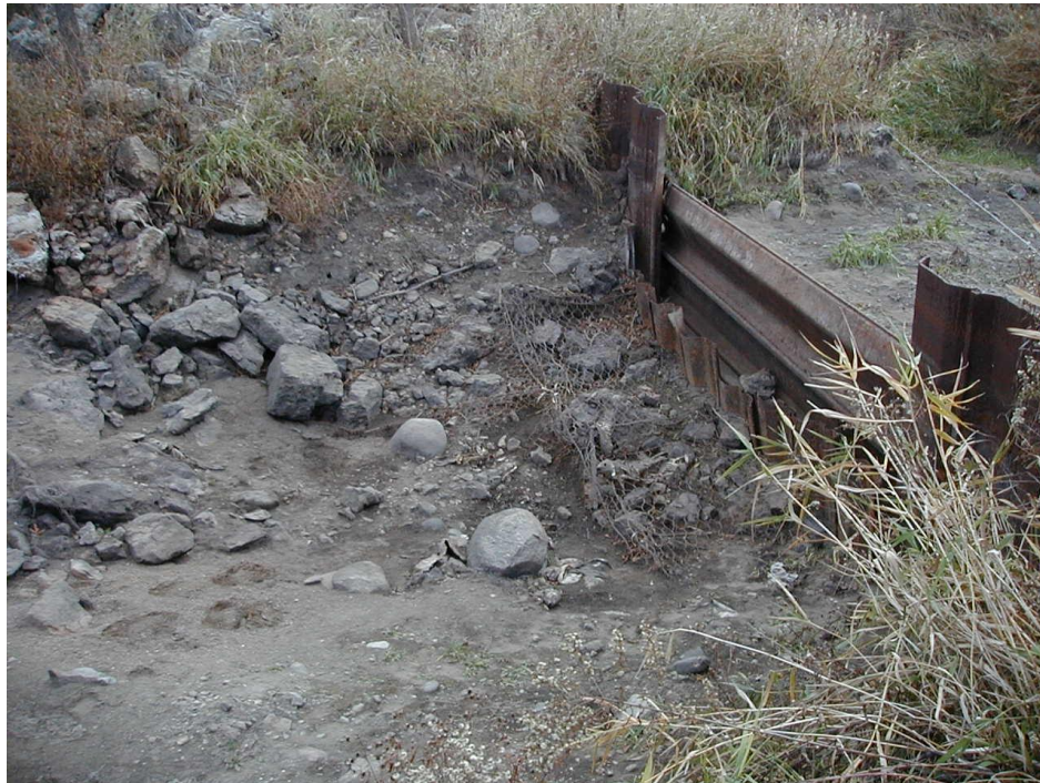
Sheet pile energy drop structure in good condition Segment 7.
