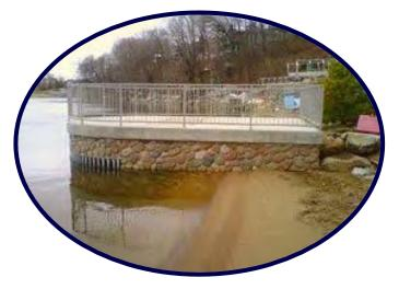
**PURPOSE:** Prior Lake is a naturally landlocked basin that is volume sensitive. The outlet structure is designed to allow water to flow out of Prior Lake during times of high lake levels in order to minimize the effects of flooding on structures around Prior Lake. Monitor the level of Prior Lake on the District's website at: www.plslwd.org/waterbodies
