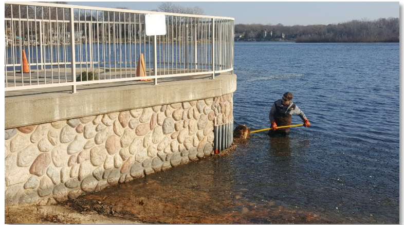
FIGURE 2 - REMOVING VEGETATION FROM OUTLET STRUCTURE
