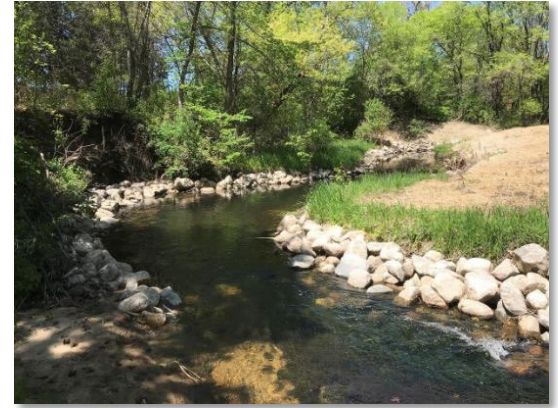
FIGURE 10 - BOULDER TOE BANK STABILIZATION IN SEGMENT 7A
