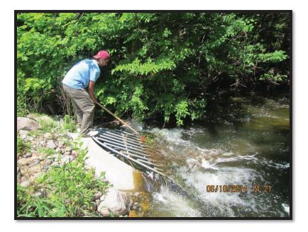
FIGURE 19 REMOVING VEGETATION FROM CULVERT GRATE AT CR42
