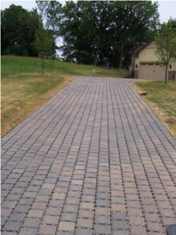
Pervious pavers at a local site.
